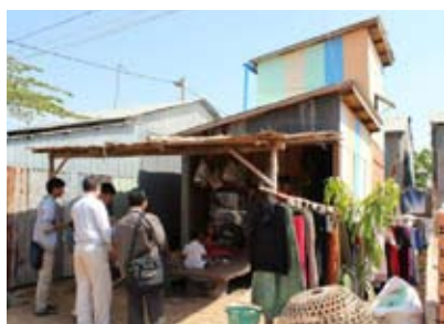
Wet + Dry House Cambodia
