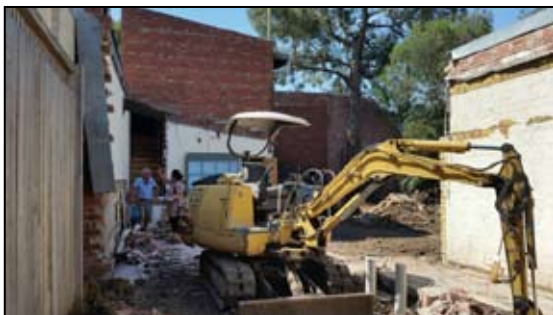
Above: Demolition continuing. Removing concrete slabs on concrete slabs .....
