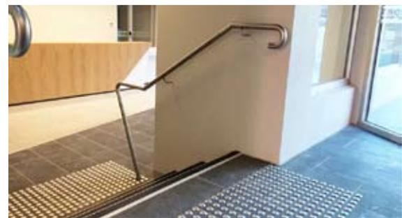
*Tactile Indicators, stair nosing, handrail extension and stairs inset from wall element provides tolerance for error when using these stairs.*
